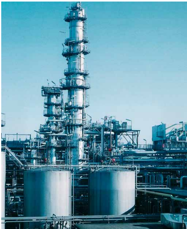
Safe and integrated power distribution with flexible application options for industrial plants.
