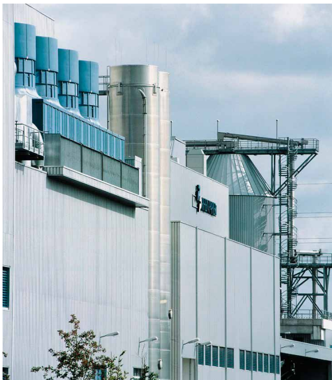
The in-line system is particularly well-suited to applications with numerous cable branches in a very confined space.
