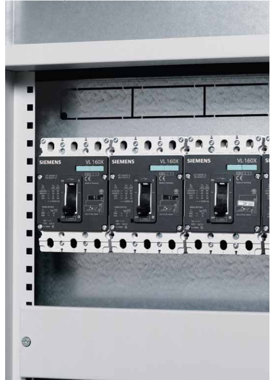
Arrangement of devices as single or multiple feeders possible.
